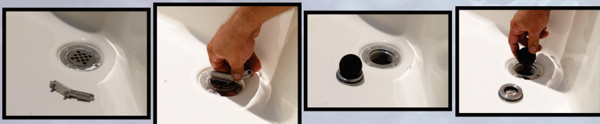
Cock Pit Drain
